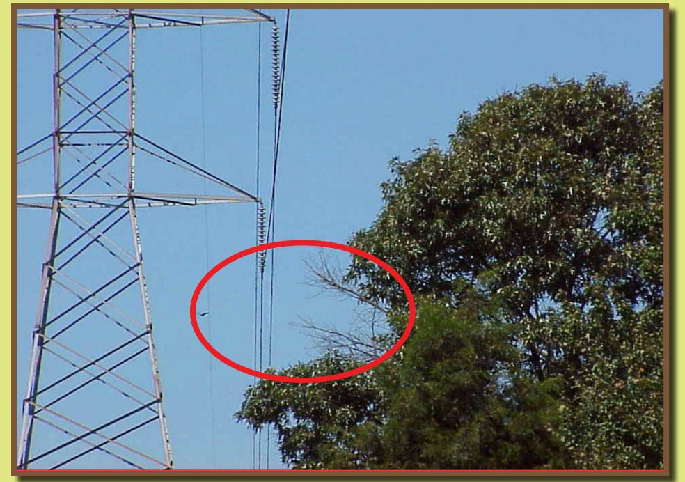
Arcing can occur even when no direct contact is made
